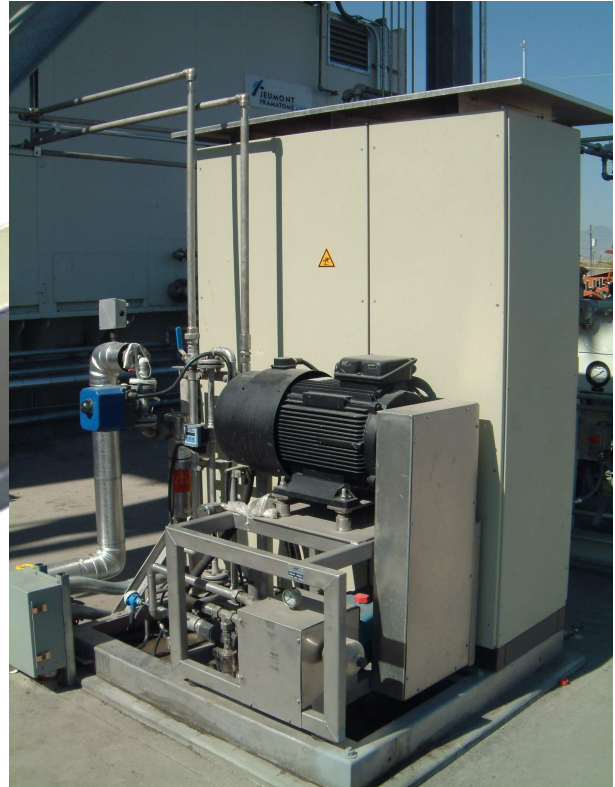
Field installation of fogging system for GE LM 6000 gas turbine (1.0 kg/s)
